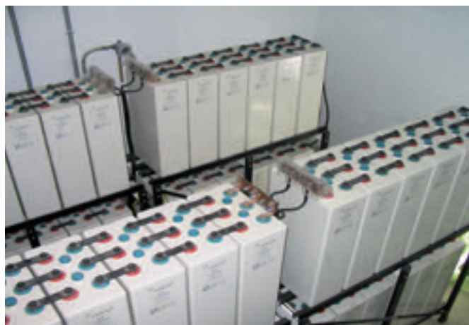
Solar photovoltaic industrial system
